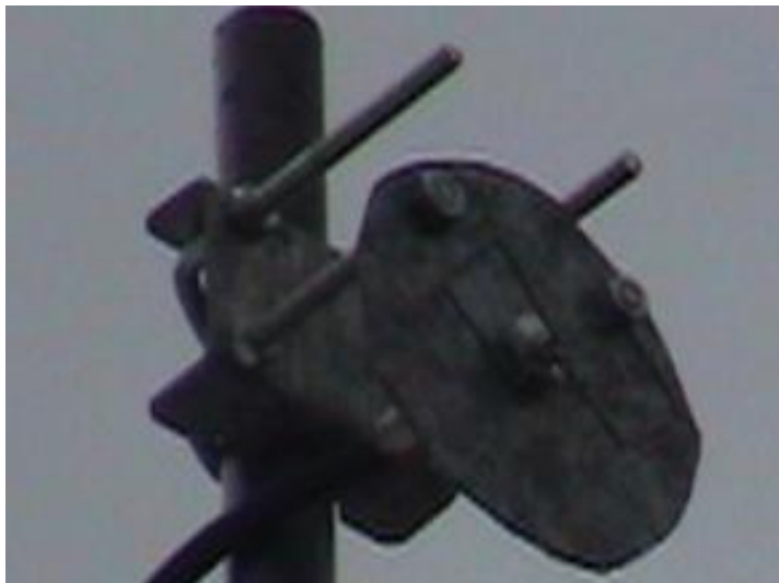
The antenna mounted on the U-bolt assembly.
